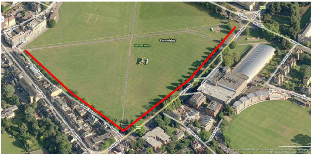
Figure 26: Bird's eye-view from BingMaps showing Parkers Piece with indicative DH pipe route on soft-ground (partial network shown) along Regent Terrace and Gonville Place
