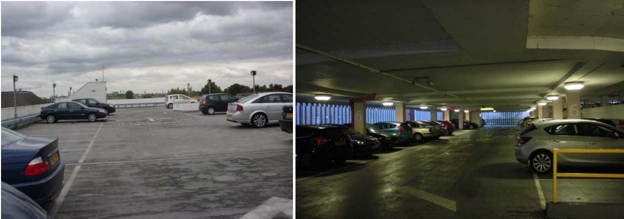
Figure 16: Photos showing the top level of the KK/QAT and a typical intermediate floor
